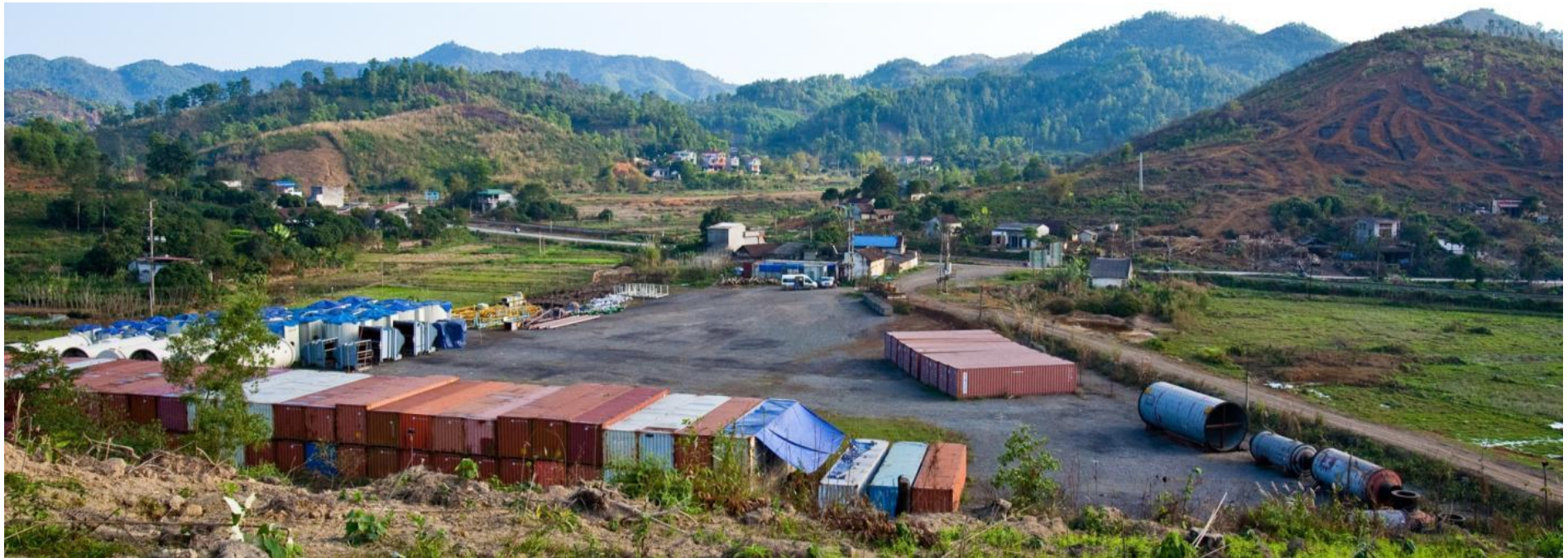
Processing Plant Equipment at the Processing Plant Site
