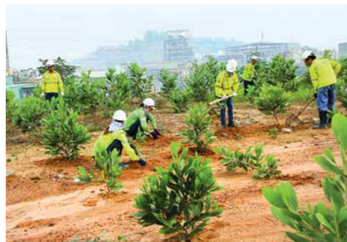
Rehabilitation work in the Nui Phao mine
