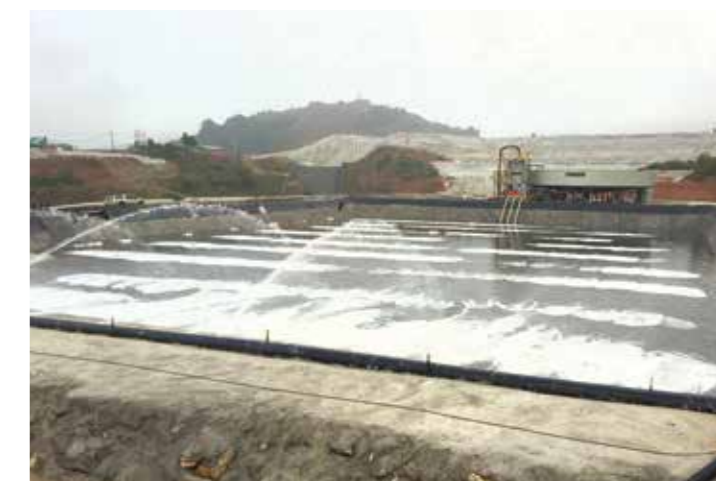
The Waste-water treatment plant in the Nui Phao mine
