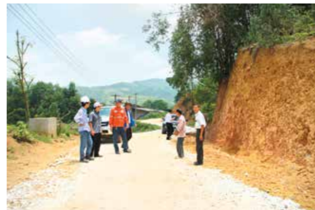
A further amount of VND 511 million was spent on upgrading 1.8km of a road in Tan Linh commune
